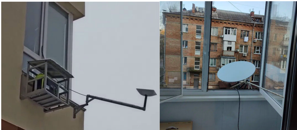
Figure 8. Examples of antenna installation of Starlink stations in cities of Ukraine (photo by https://highload.today ).
